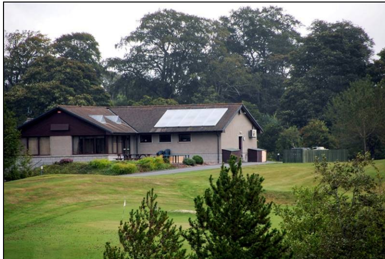
Solar panels on clubhouse roof
